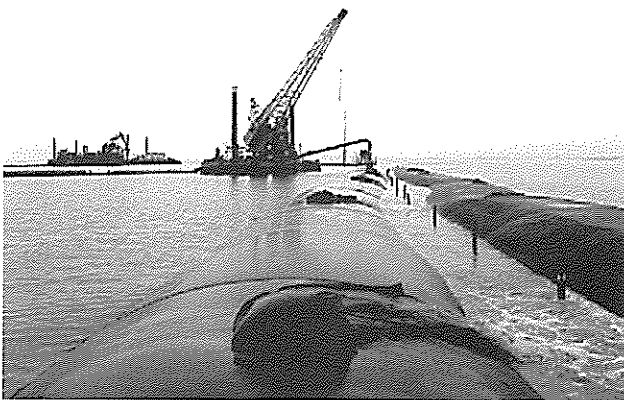
c) Filling of geotextile tubes
